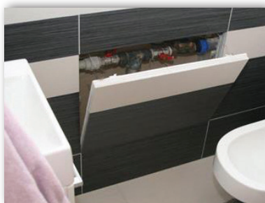
Installed door – virtually invisible
